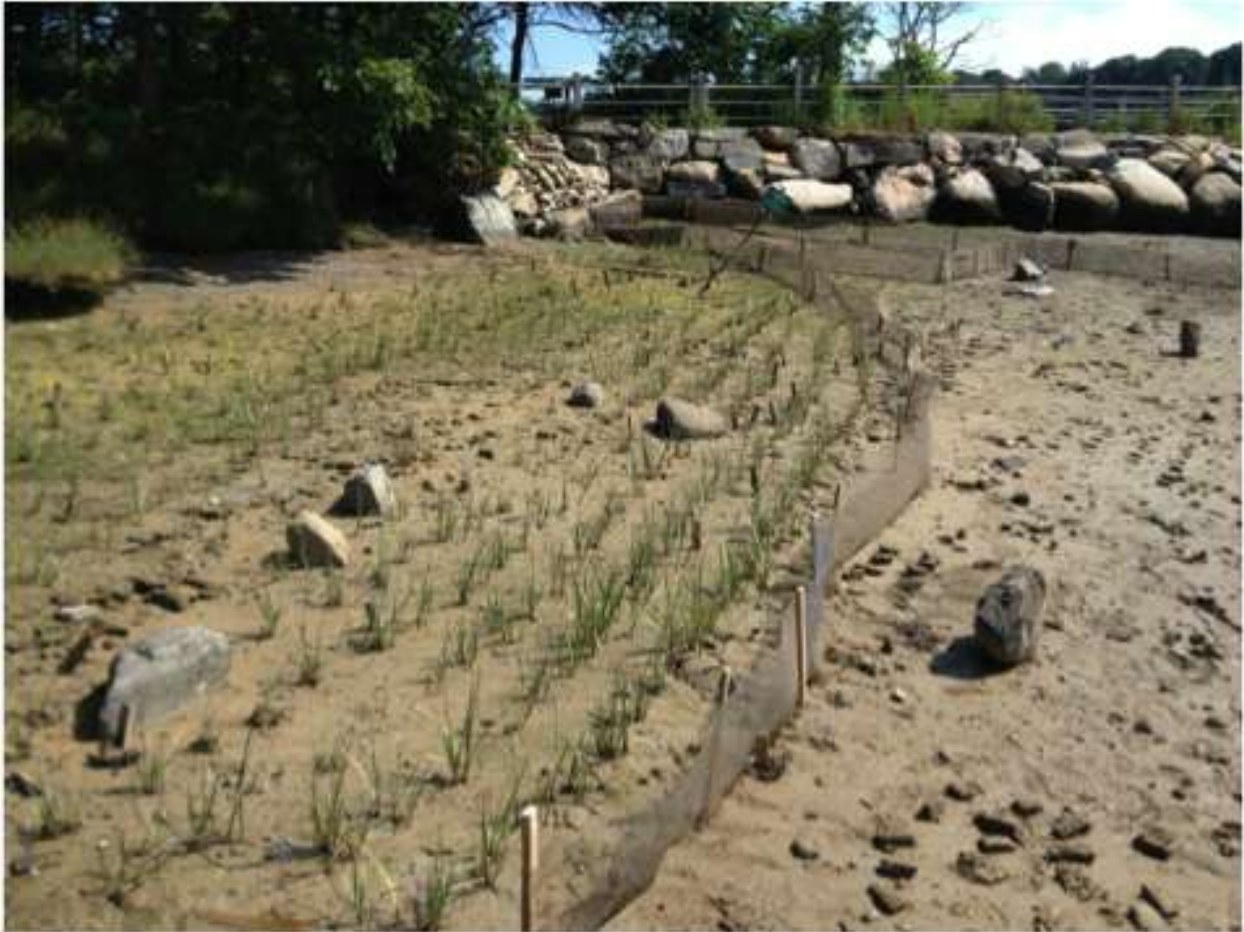
Figure 7. Restoration along the York River shoreline in July, 2017.
